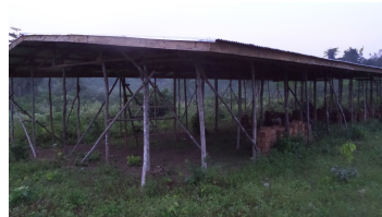
New school building under construction
